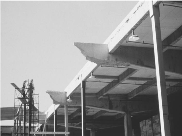
*Figure 1.3: Picture of the shear failure of roof beams in Air Force Warehouse, Ohio, August 1955.*
